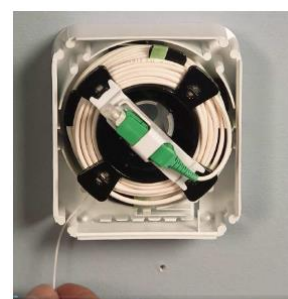
Step 3: Spool out the 900um fiber
