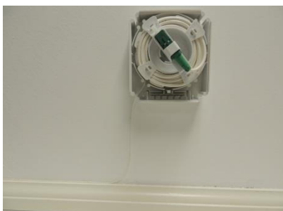
Micro-drop adhered to the wall near the module. Rotate the spool to take up remaining slack and adhere to the entry point.
